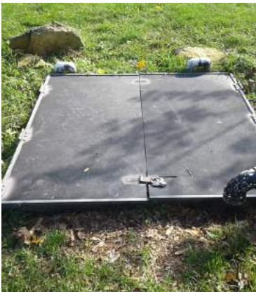
Pump vault door
