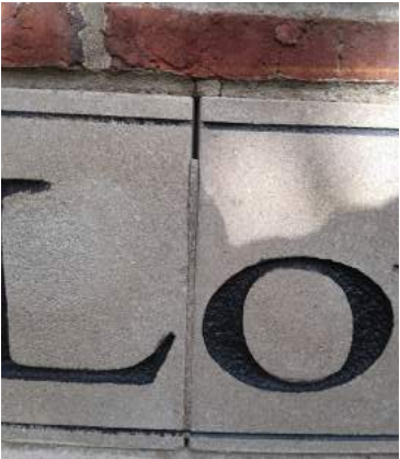
Entry sign mortar
